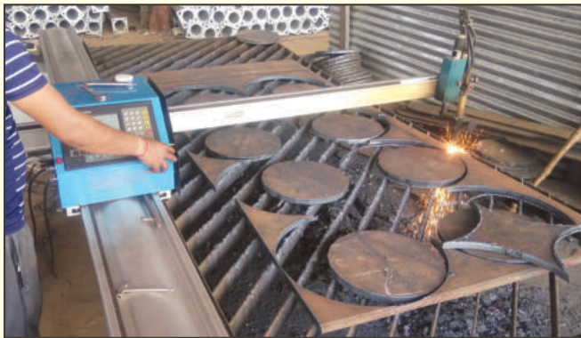
BASE PLATE CUTTING
