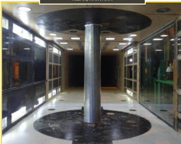
NATIONAL WIND TUNNEL FACILITY
