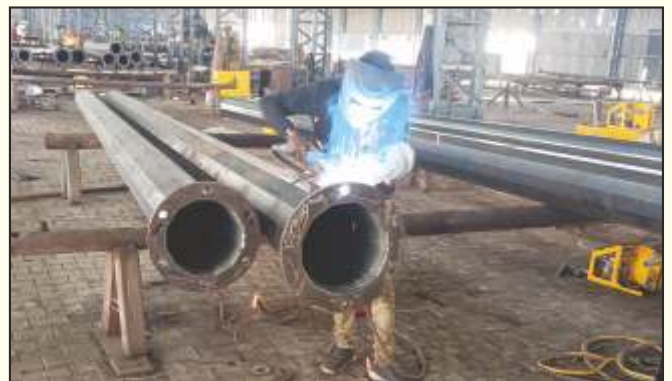
BASE PLATE FABRICATION
